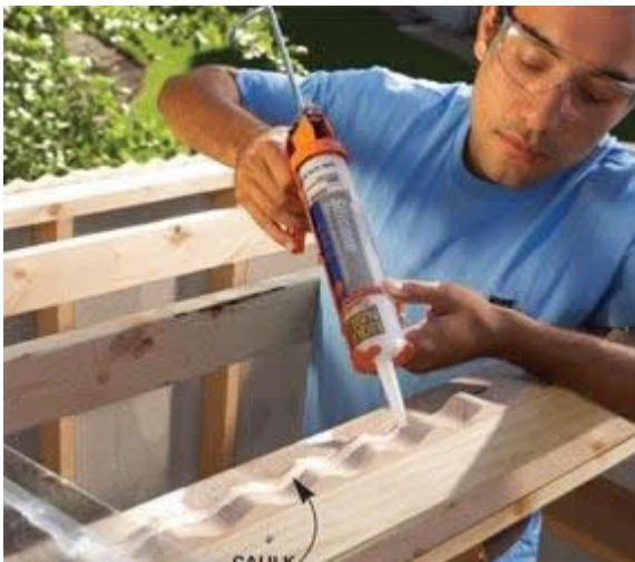
PHOTO 8: ADD THE ROOF PANELS
